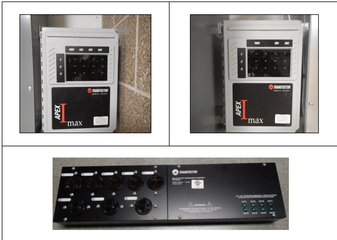
Figure 7: Surge Protection Devices: Type I (left), Type II (right), and Type III (bottom)
