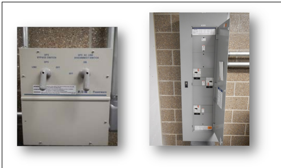
Figure 5: Bypasses: Make-before-break (left) and Online Double Conversion (right) 52
