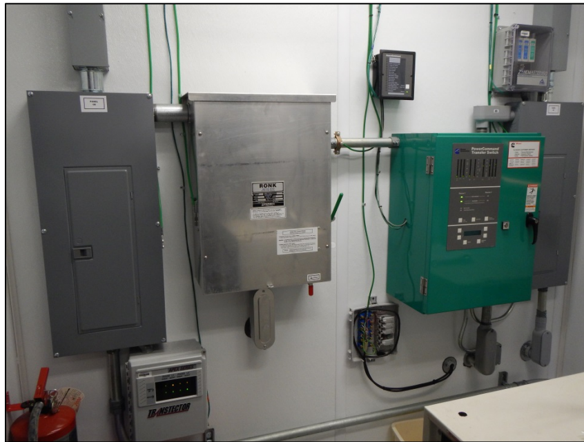
Figure 3: Power System with Automatic and Manual Transfer Switch
